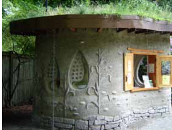
Stanley Park Cob House (Photo: SPES)
